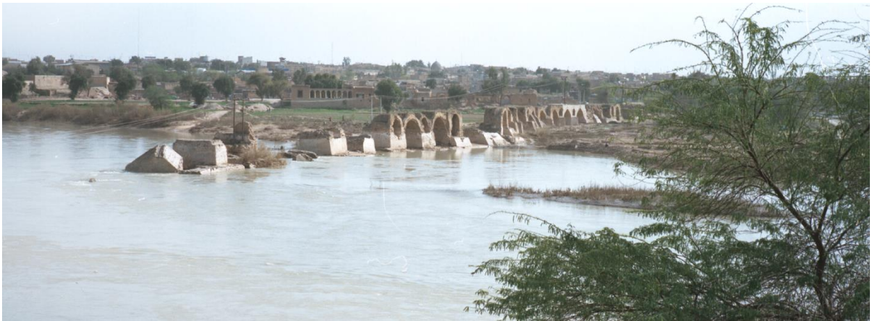
Figure 2.27 The southern arches are very poorly preserved and at the same time significantly modified through intrusive renovations.
