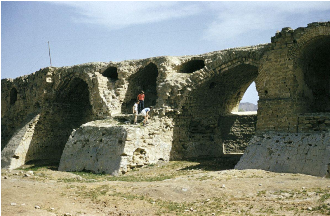
Figure 2.53. Recent restorations in the southern part of the Shadorwan have affected the authenticity of the monument. In particular, the heterogeneity of the shape and size of the arches is completely covered hidden under the renovated façade. Top, south arches in 1958-59. (Photo taken by Charles Schroeder, copyright, Harvard Fine Arts Library, Special Collections. Bottom, south arches in 2004.
