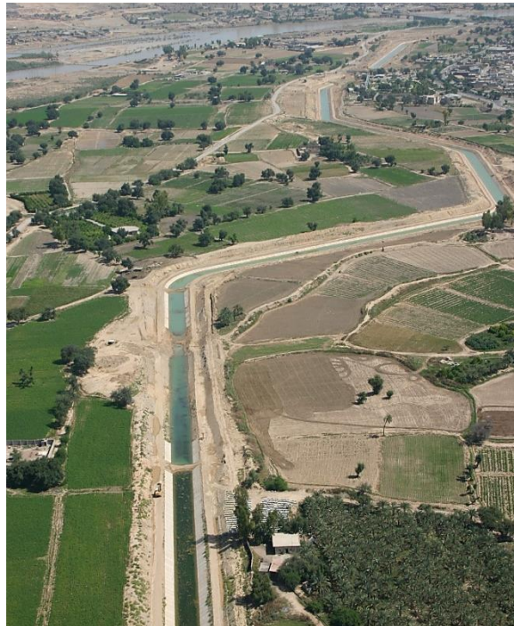
Figure 2.16 Main channel of the Dariun after renovation: a cement canal replaced the old channel.
