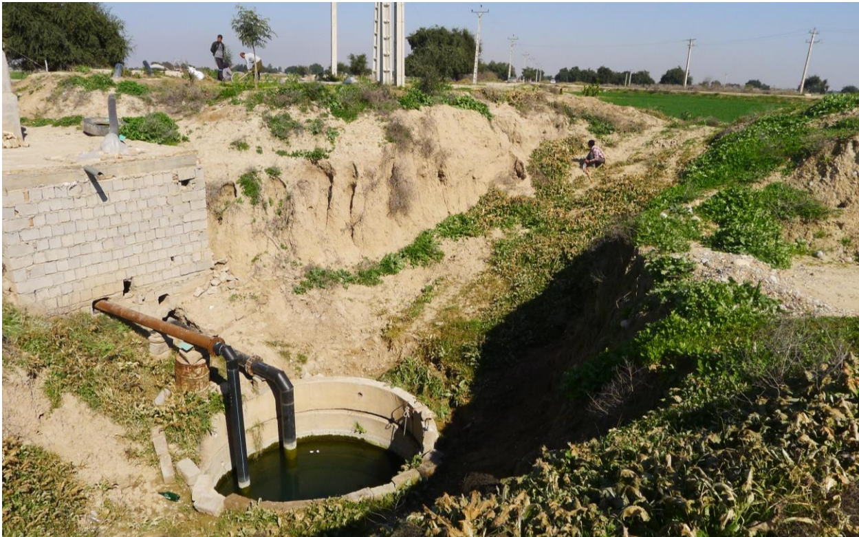
Figure 5.14. A modern canal passing to the east of KS1812 is nonfunctional because of design error. Instead, water from the well excavated at KS1812 is pumped in the old canals to supply the nearby fields.
