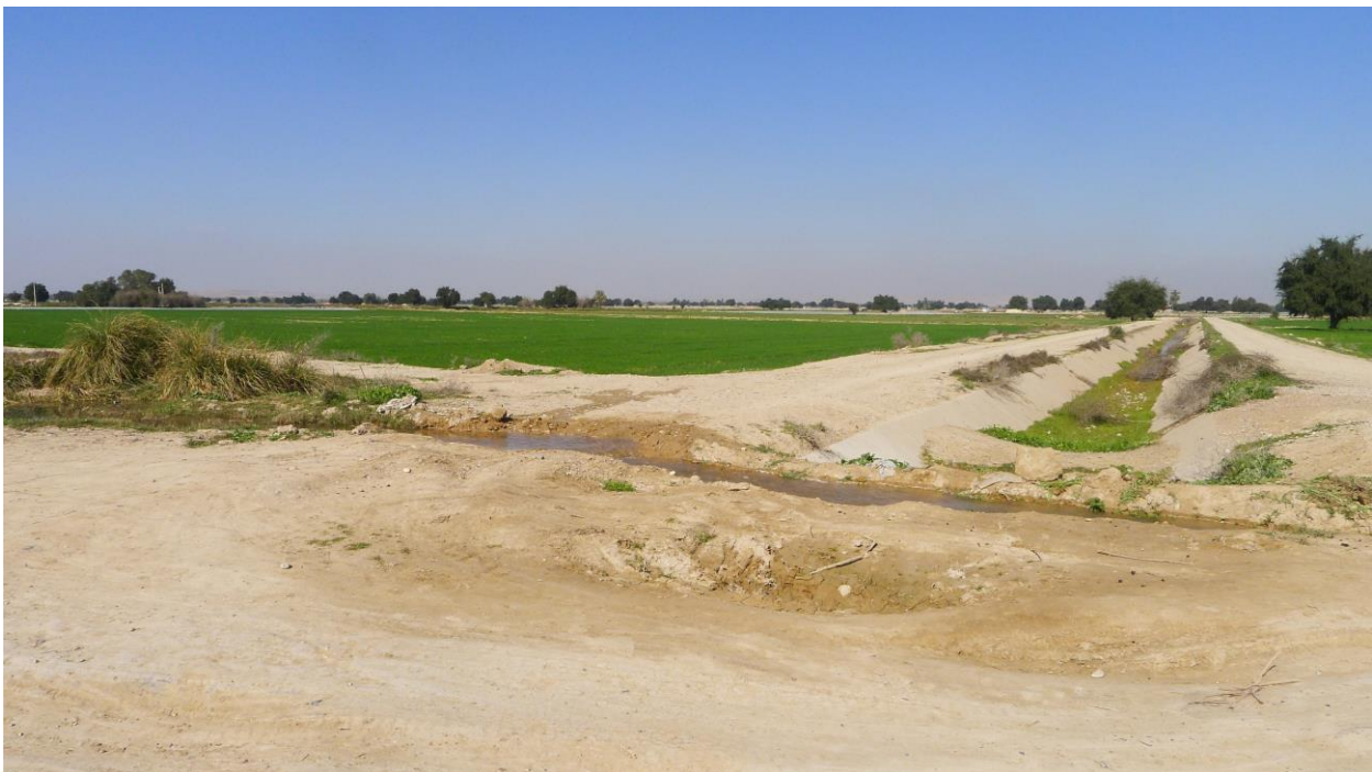
Figure 5.14. A modern canal passing to the east of KS1812 is nonfunctional because of design error. Instead, water from the well excavated at KS1812 is pumped in the old canals to supply the nearby fields.
