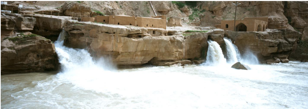
Figure 2.30 The southern face of the Gargar Dam. The sloping part and two phases of the straight wall are visible on the image. To the left are the additional buildings of the Pahlavi period.
