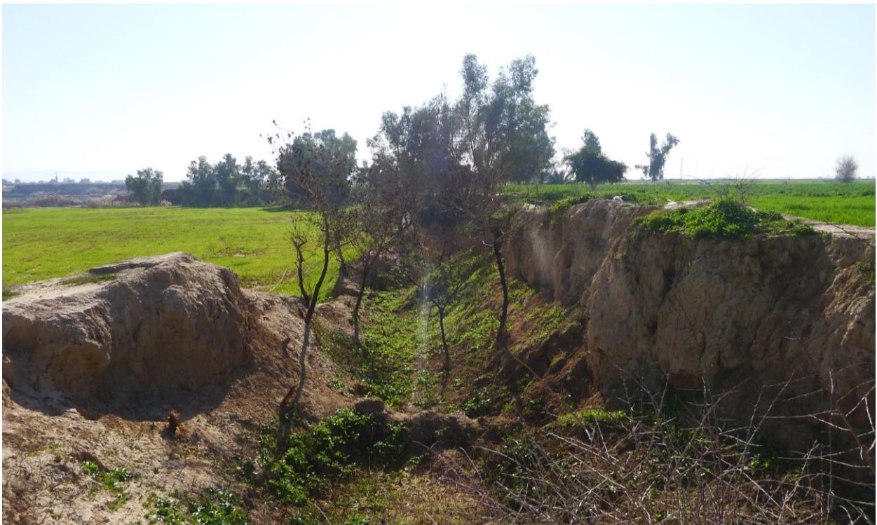
Figure 5.20 The south end of the above canal, destroyed as a result of water erosion along the Gargar valley.
