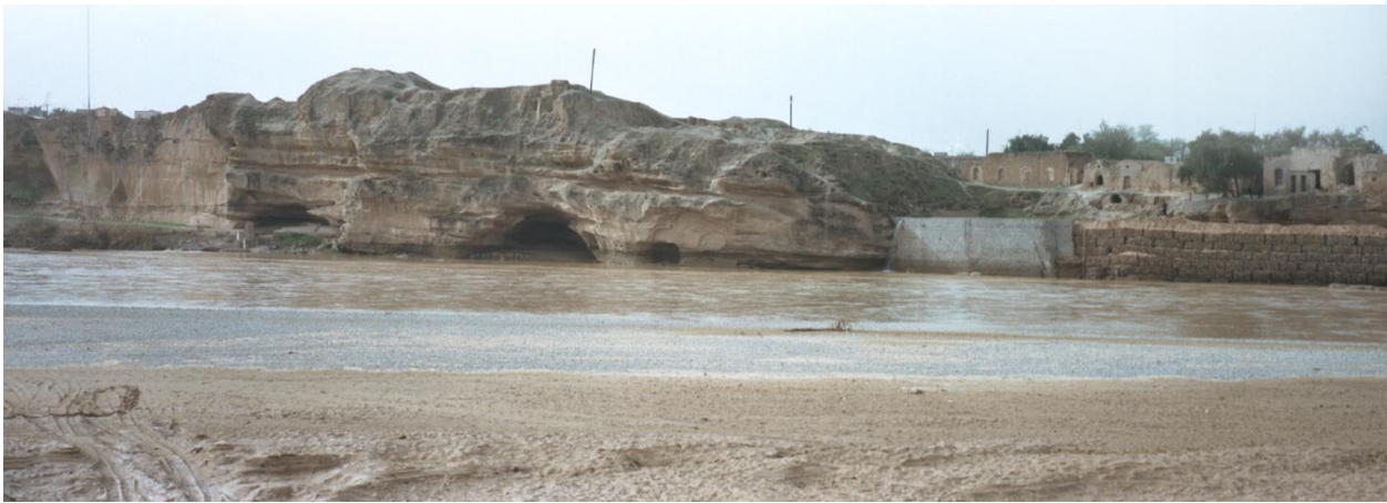
Figure 2.17 The old intakes of Dariun beneath the Salasel Castle; To the right: new intake that replaced the main headwork of the canal.
