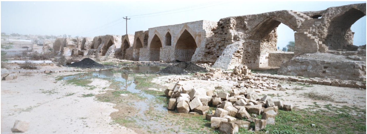
Figure 2.27 The southern arches are very poorly preserved and at the same time significantly modified through intrusive renovations.
