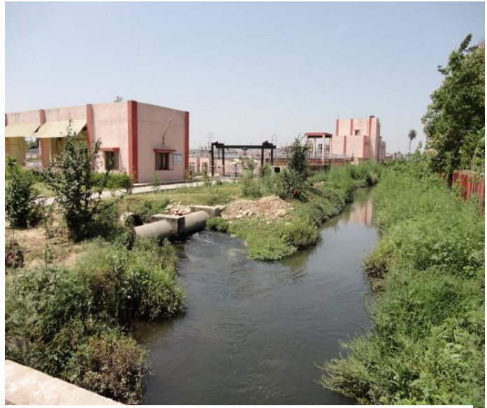
Picture 24: Image of Jagjeetpur drain at Haridwar
