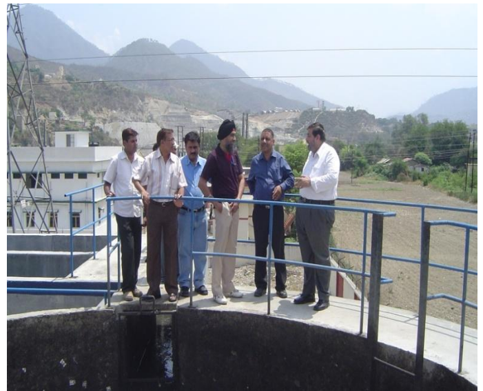
Picture 15: STP at Sringar
