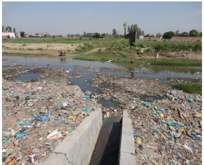
Picture 28: Malan river at Nazibabad (Bijnore)
