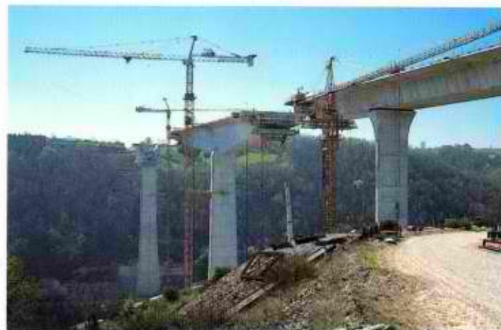
The Tanus viaduct, over the Vaur, was built by Dodin. Its central span measures 190 meters.
