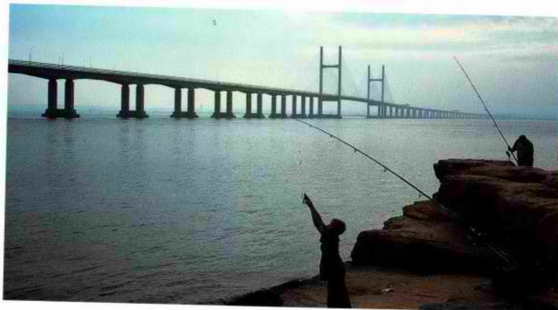
The second bridge of the River Severn. Freyssinet performed hoisting operations, the pre-stressing for the masts and diaphragms, and installed 240 stay-cables.
