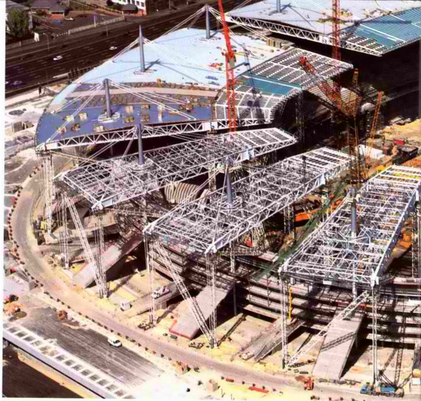
The roof of the Stade de France is held in place, 42 metres above the playing field, by eighteen tapered masts.
