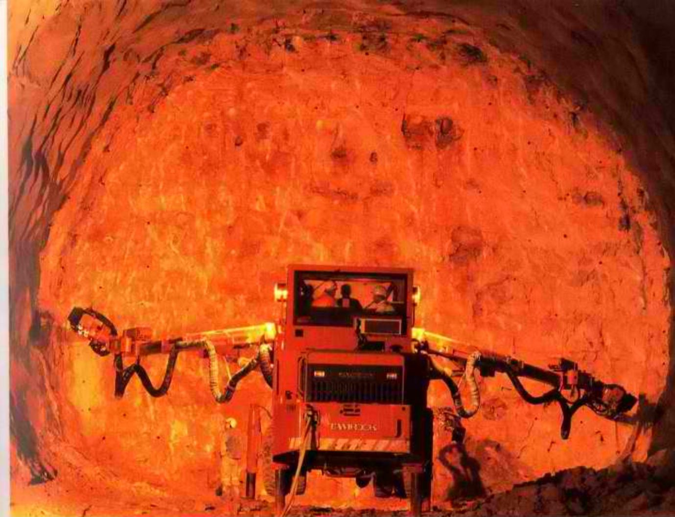
The TGV tunnel in Marseilles (5414 metres long), with its exceptional diameter, is being driven using explosives.
