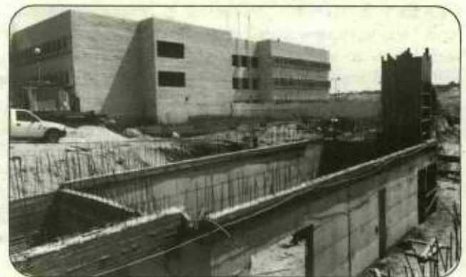
First city high school: Located in the Dekel Vilnai school and sports center complex. Building is in the first stage of construction. Expected completion date: September 1996.
