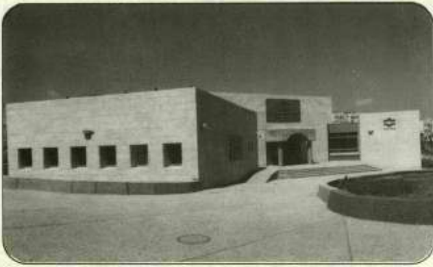
Kupat Cholim Clalit. Construction completed. Mother & Child health clinic on first floor, Kupat Cholim Clalit medical center on second floor.
