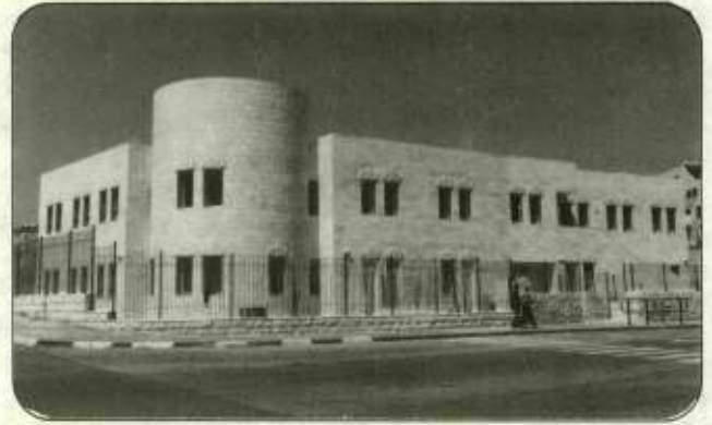
Kupat Cholim Leumit. Construction completed. Kupat Cholim Leumit medical center. A section of the building is used by the Nili daycare center.
