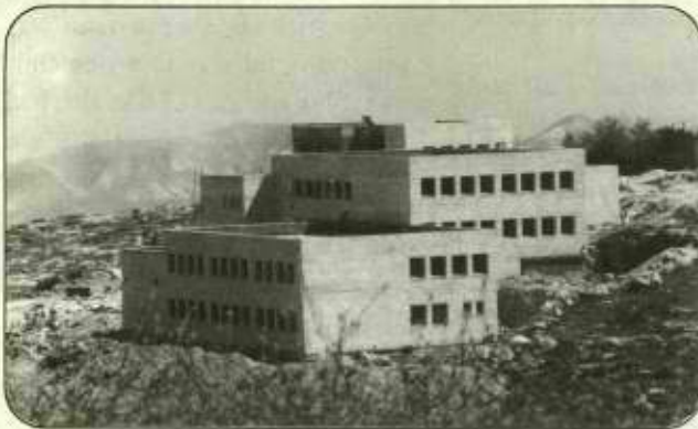
Ma'ale Hatorah elementary school: Located in the new educational complex near the city nursery. Building in progress. Expected completion date: September 1995.
