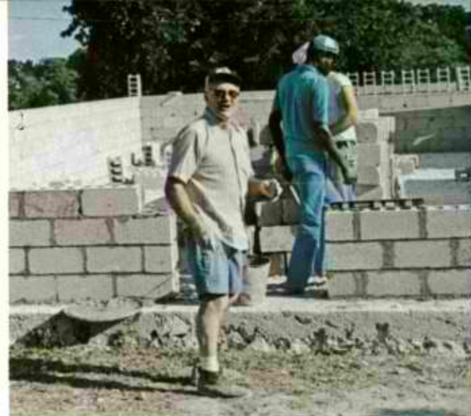
As needs arise, we send technical personnel to provide specific services on mission fields. This American businessman oversees construction of a memorial library in Haiti.
