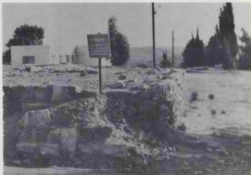
ALL THAT IS LEFT OF NEVE OVADIA IN THE PRESENT DAY KIBBUTZ ARE ITS FOUNDATIONS, PHOTOGRAPHED AT KIBBUTZ KFAR ETZION IN 1969.
