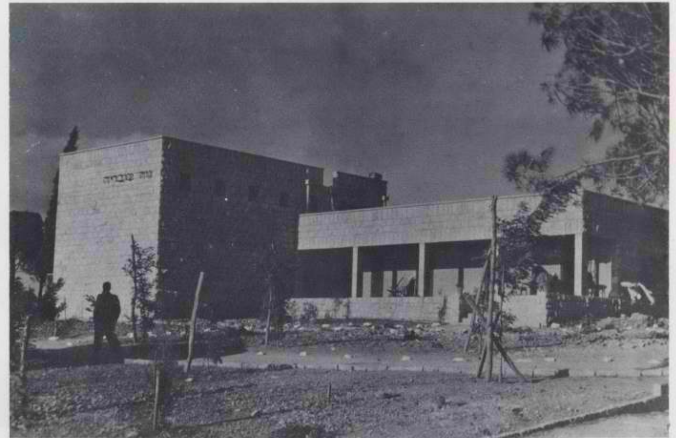
"NEVE OVADIA." The destroyed cultural center of the old Kibbutz of 1948. ABOVE NOW. Bulldozers and workmen building the new village center at Gush Etzion. (The Lonely Tree - upper right.)
