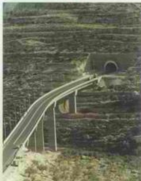
Tunnel Road to Eilat
