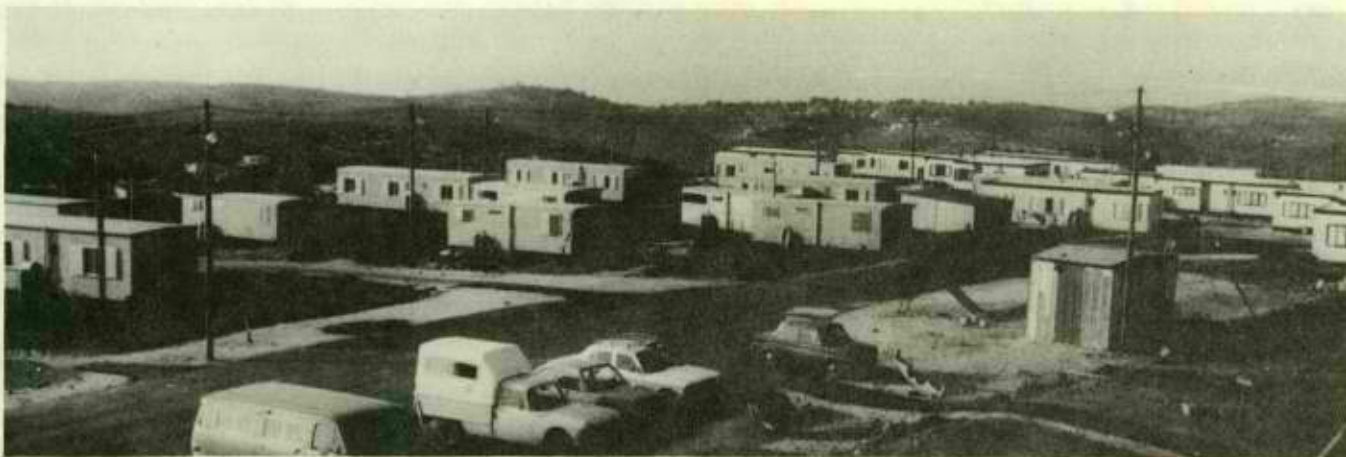
General View of prefabs
