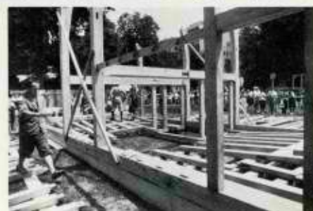
Craftsmen using seventeenth-century style tools and techniques assist in the raising of a replica of the Fairbanks House of 1630.
