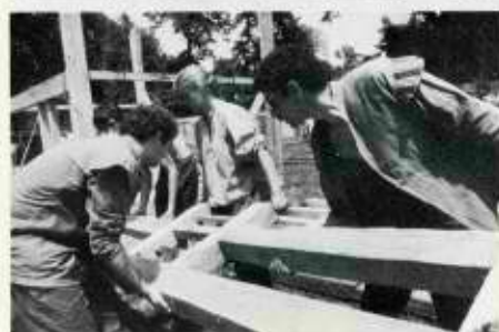
Craftsmen using seventeenth-century style tools and techniques assist in the raising of a replica of the Fairbanks House of 1630.
