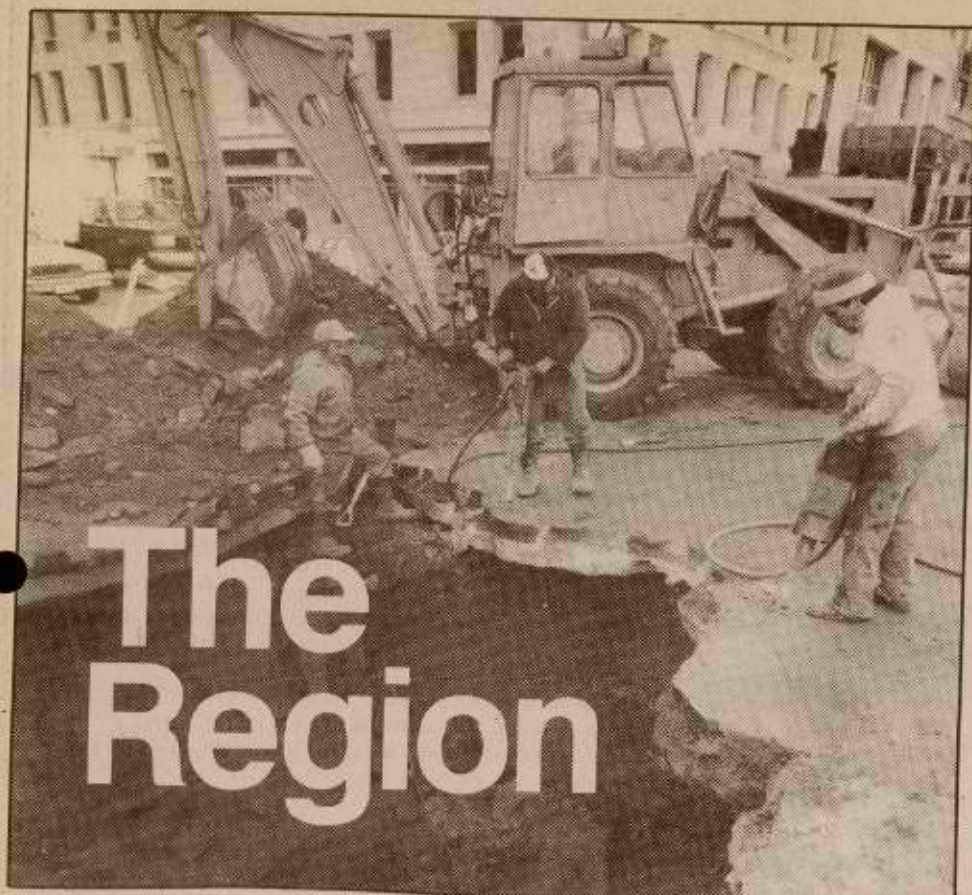
Emergency work on a broken water main.
