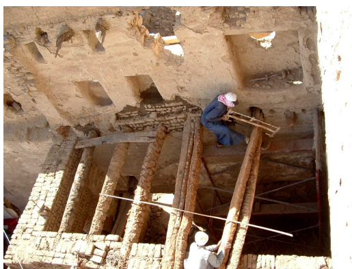
Figure 44 Putting floor beams for the first floor of BQur 1.
