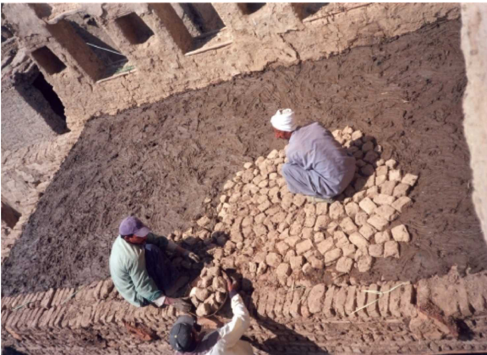
Figure 50 Putting on the top layer of the second floor of BQur 1.
