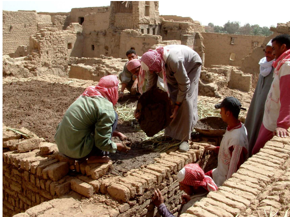
Figure 46 Laying the mud layer for the first floor of BQur 5.
