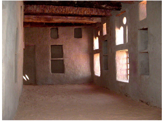
Figure 40 Newly plastered hall on the second floor of Bayt al-Qadi.
