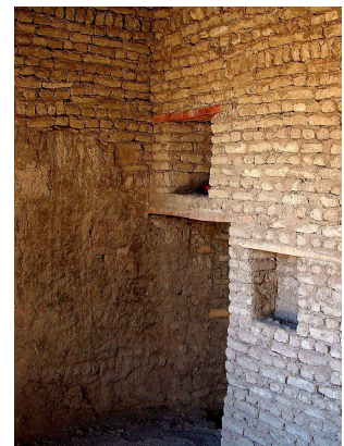
Figure 43 Rebuilt wall between BQur 2 and 5.
