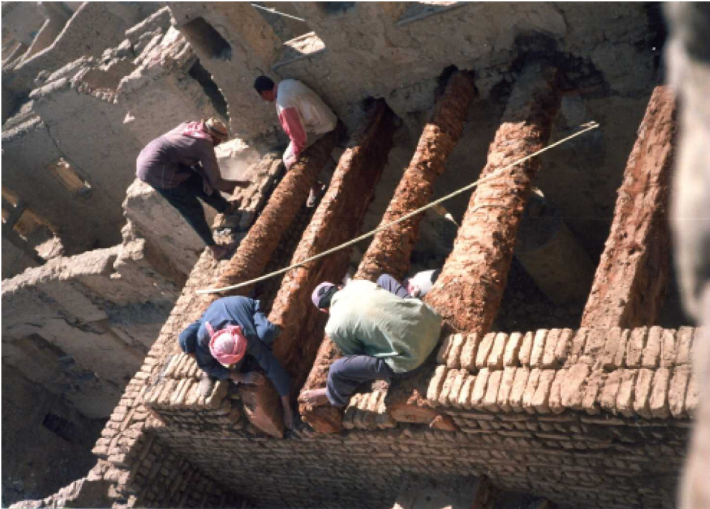
Figure 49 Putting floor beams for the second floor of BQur 1.
