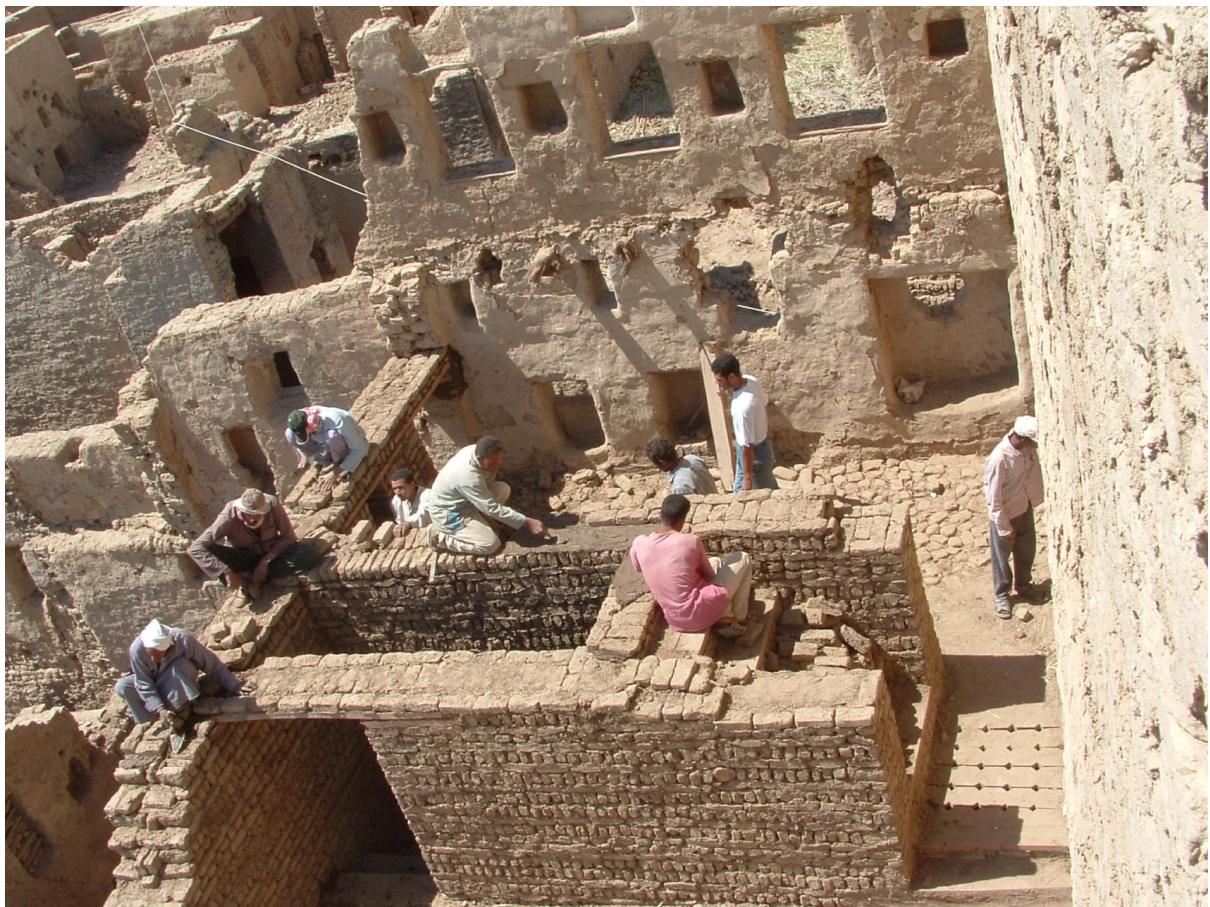
Figure 48 Reconstructing the walls on the first floor of BQur 1.
