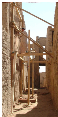
Figure 41 Shoring up of the façade of Bayt al-Qurashi.
