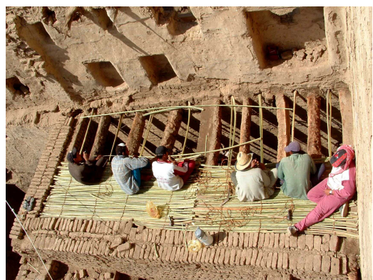
Figure 45 Laying the palm nerves for the first floor of BQur 1.
