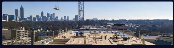
First mass-timber office project in Atlanta; ~205,000 SF built of DLT over glulam with steel bracing
