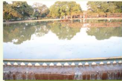
Clarification tank of Okhla Sewage Treatment Plant (STP)
